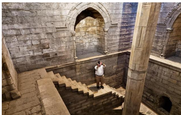
Figure 3 The Nilometer used by Ancient Egyptians to monitor the Nile River flood level (Source: Mortel 2022).
